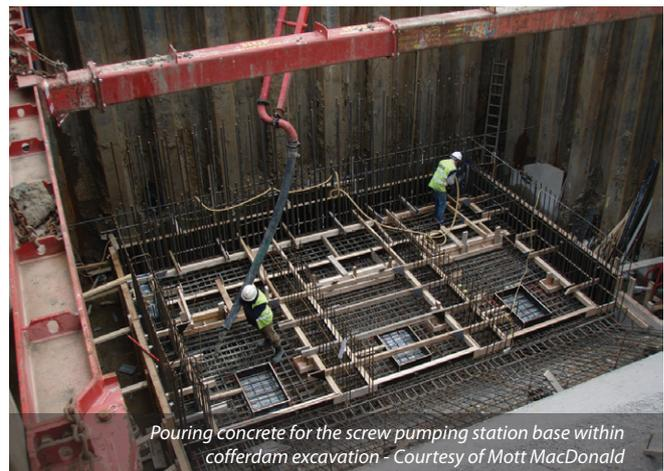
Pouring concrete for the screw pumping station base within cofferdam excavation - Courtesy of Mott MacDonald
