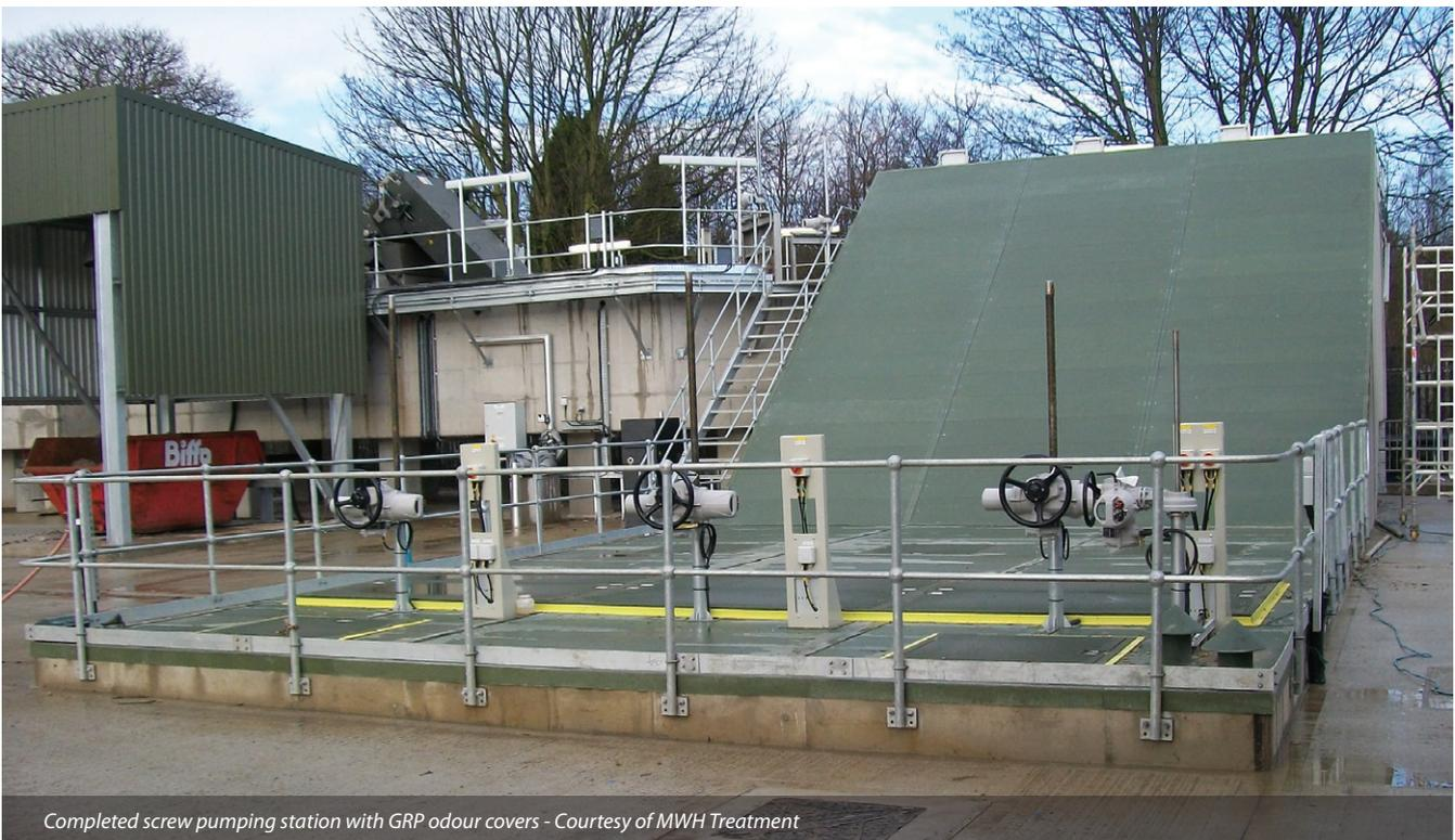
Completed screw pumping station with GRP odour covers - Courtesy of MWH Treatment
