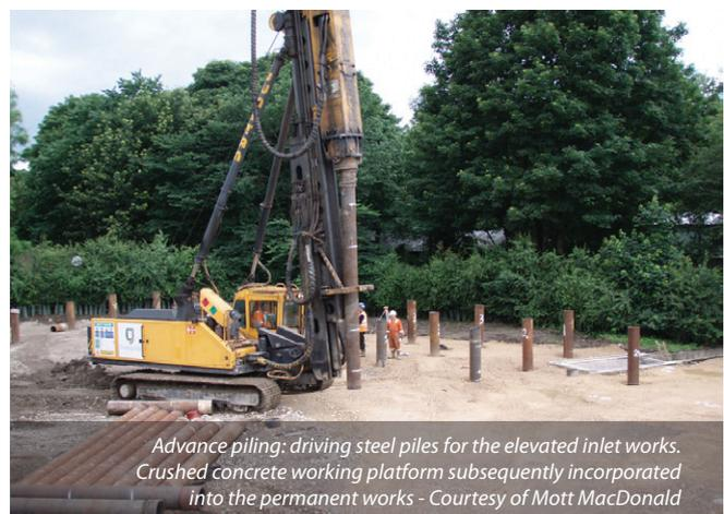
Advance piling: driving steel piles for the elevated inlet works. Crushed concrete working platform subsequently incorporated into the permanent works - Courtesy of Mott MacDonald
